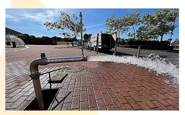
If there are any small parts required like false spindles, hydrant caps and H Plates these can be fitted during the testing to ensure the hydrants work and be identified as they should at all times. We can also paint the hydrant covers yellow should they be fading or not painted.
